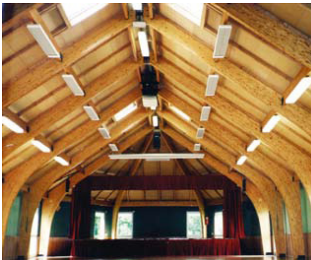
EZ gives instant heat and no preheating is necessary which makes it ideal for buildings that are used on an irregular basis.
